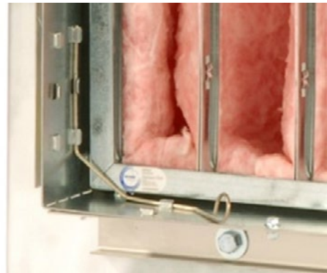
Installation af Universal Filter Holding Frame
